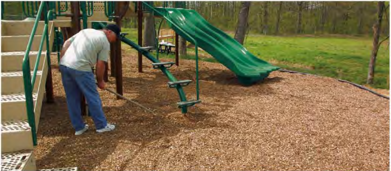
Raking loose-fill engineered wood fiber material
