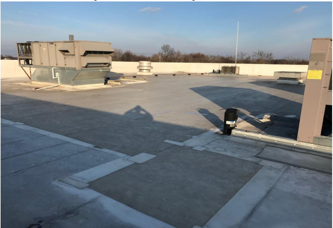
View looking north east of PVC flat roof 12-18-2018
