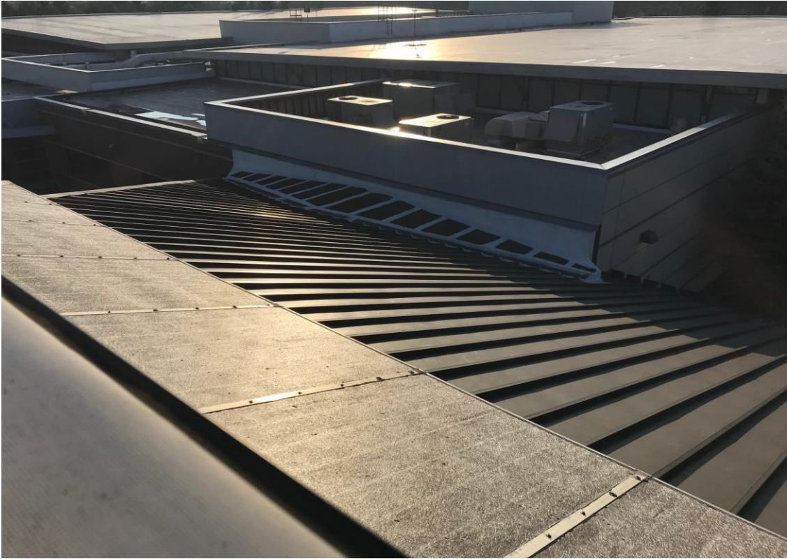
View looking west at cricket attachment to Ice Arena Addition
