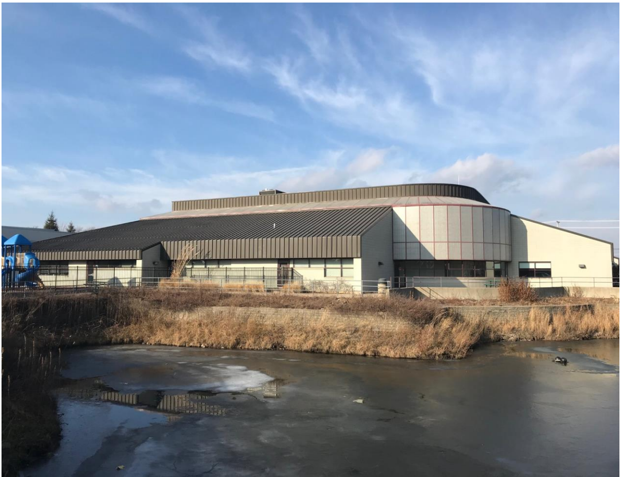
View looking north at south Building Elevation 12-18-2018
