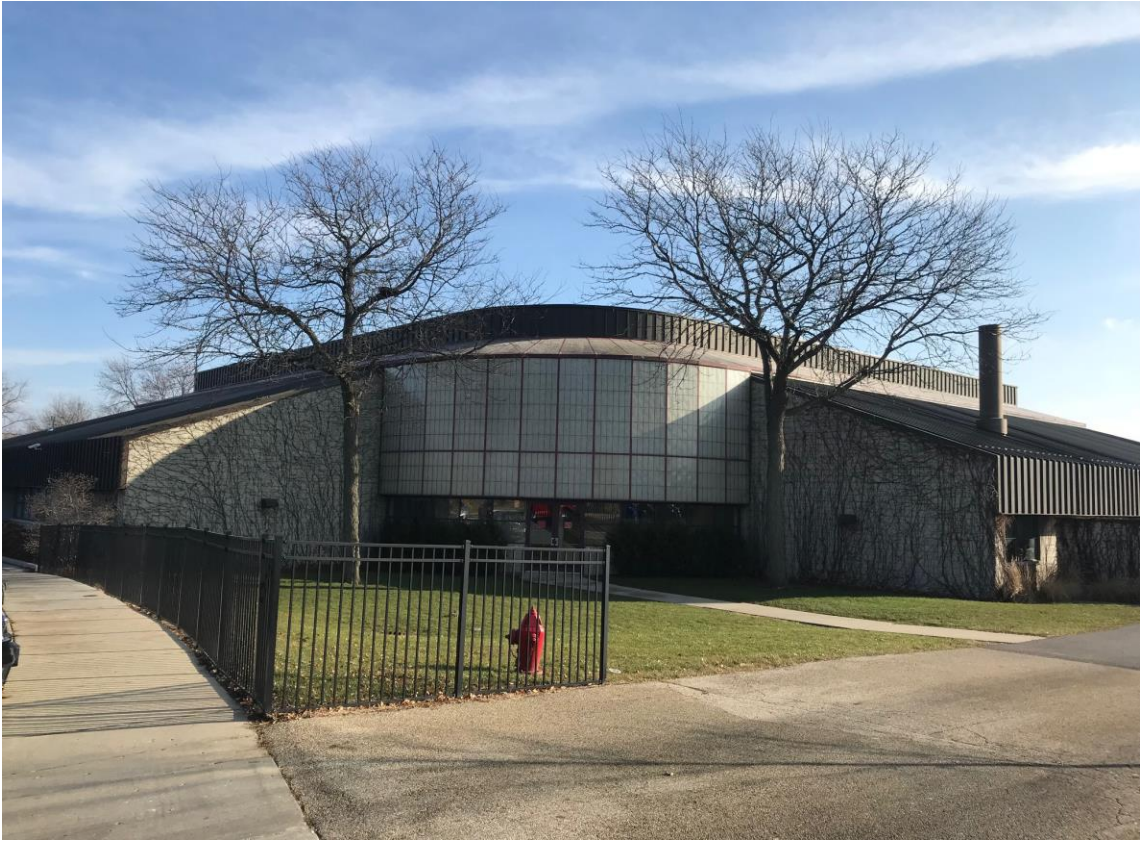
View looking south-east at North Building Elevation 12-18-2018
