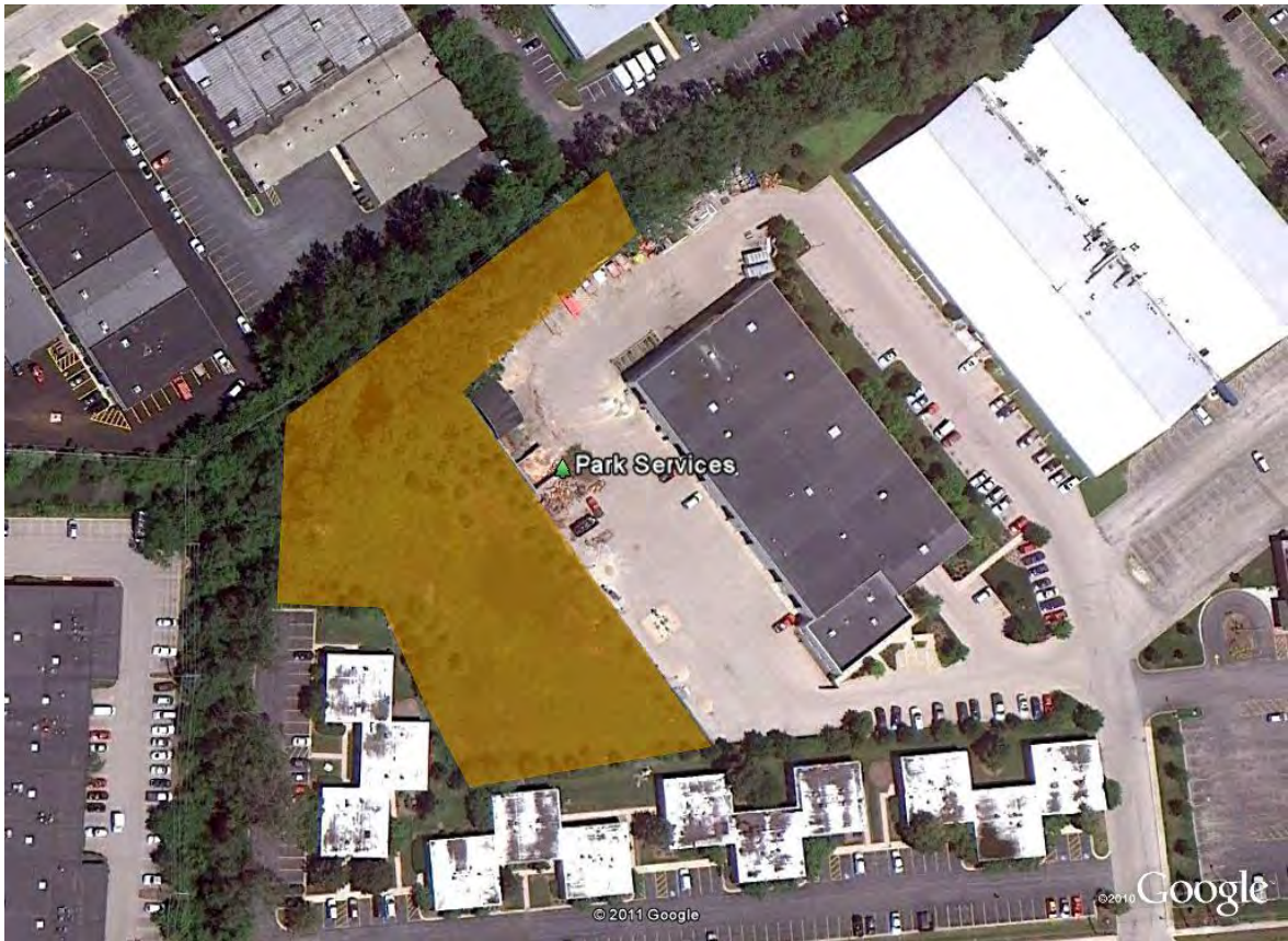
Park Services is the 4.3 acre maintenance facility and contains 1.55 acres of naturalized retention.
